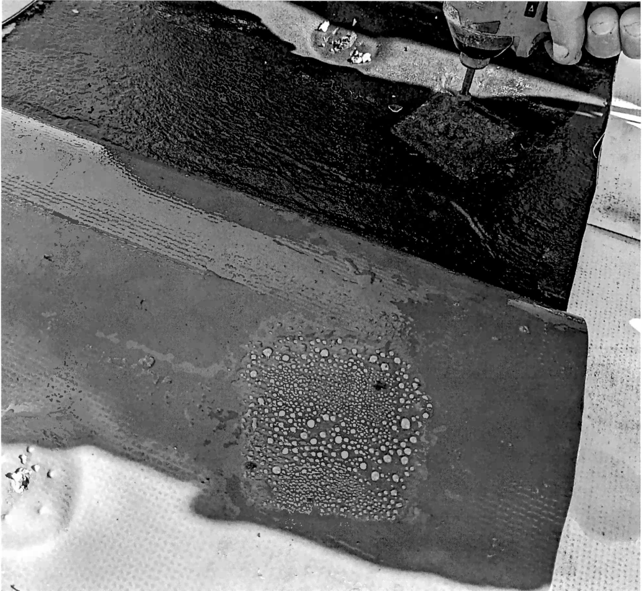
Figure 19 cut #4, another illustration of the complete saturation of materials.
