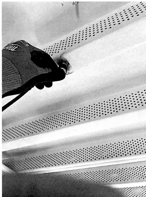
Photo-6: Ultrasonic probe on test location
