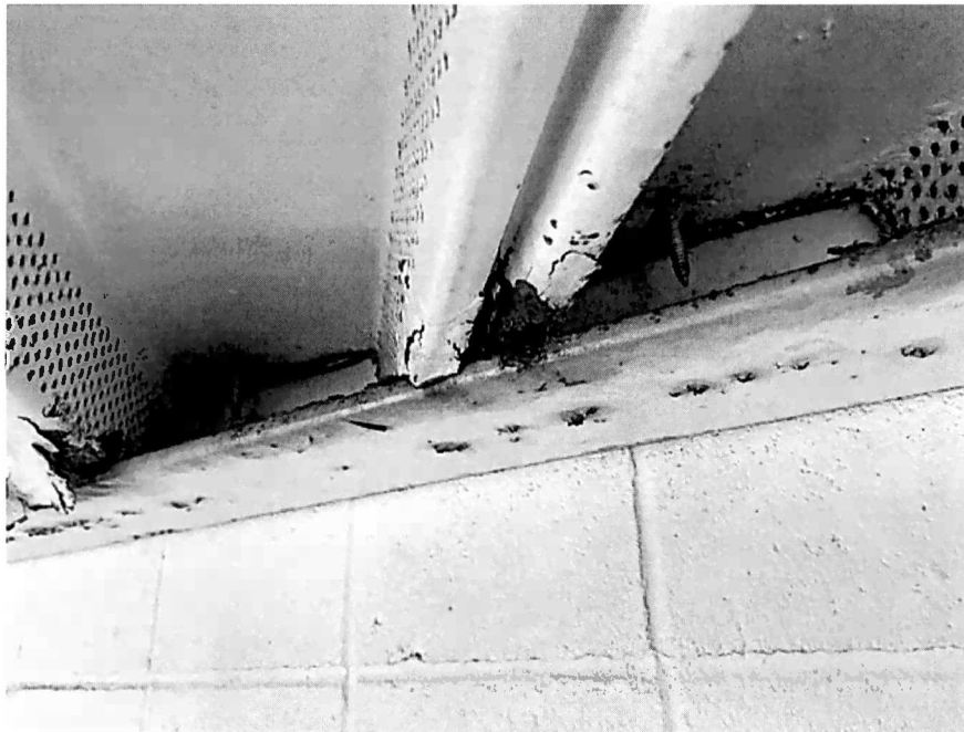
Photo-9: Settlement cracking. Unrelated to roof deck problems North corner of building
