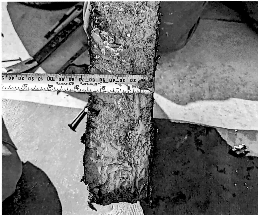
Figure 4 cut #1, first layer of 2.5-inch polyiso insulation.
