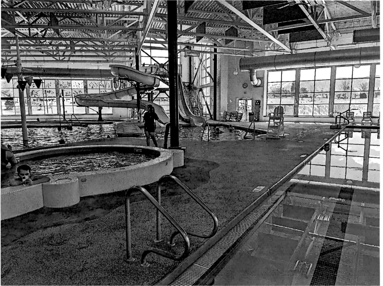
Figure 43 interior where no air flow was detected. Often found this to be an area with lifeguard activity.
