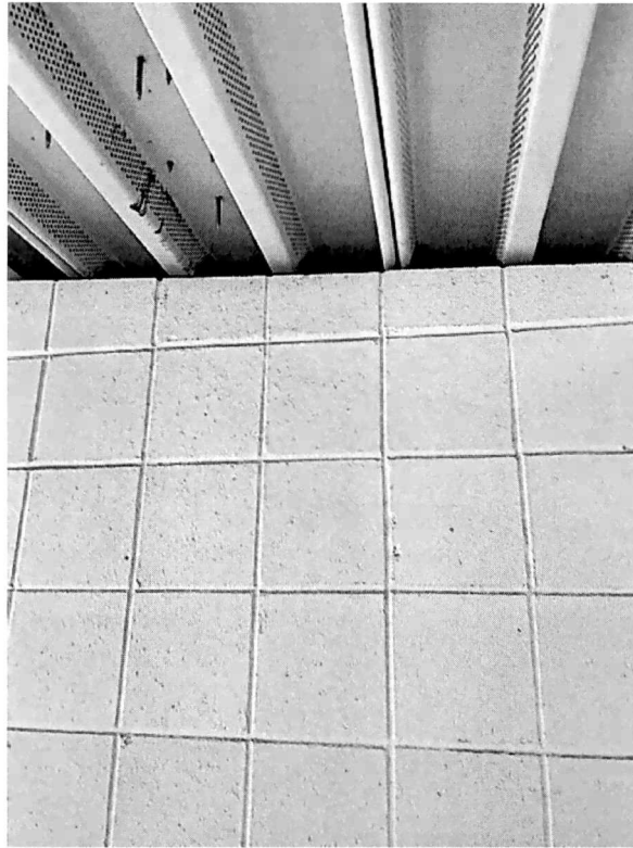
Photo-21: Lightly damaged roof deck bearing at west wall
