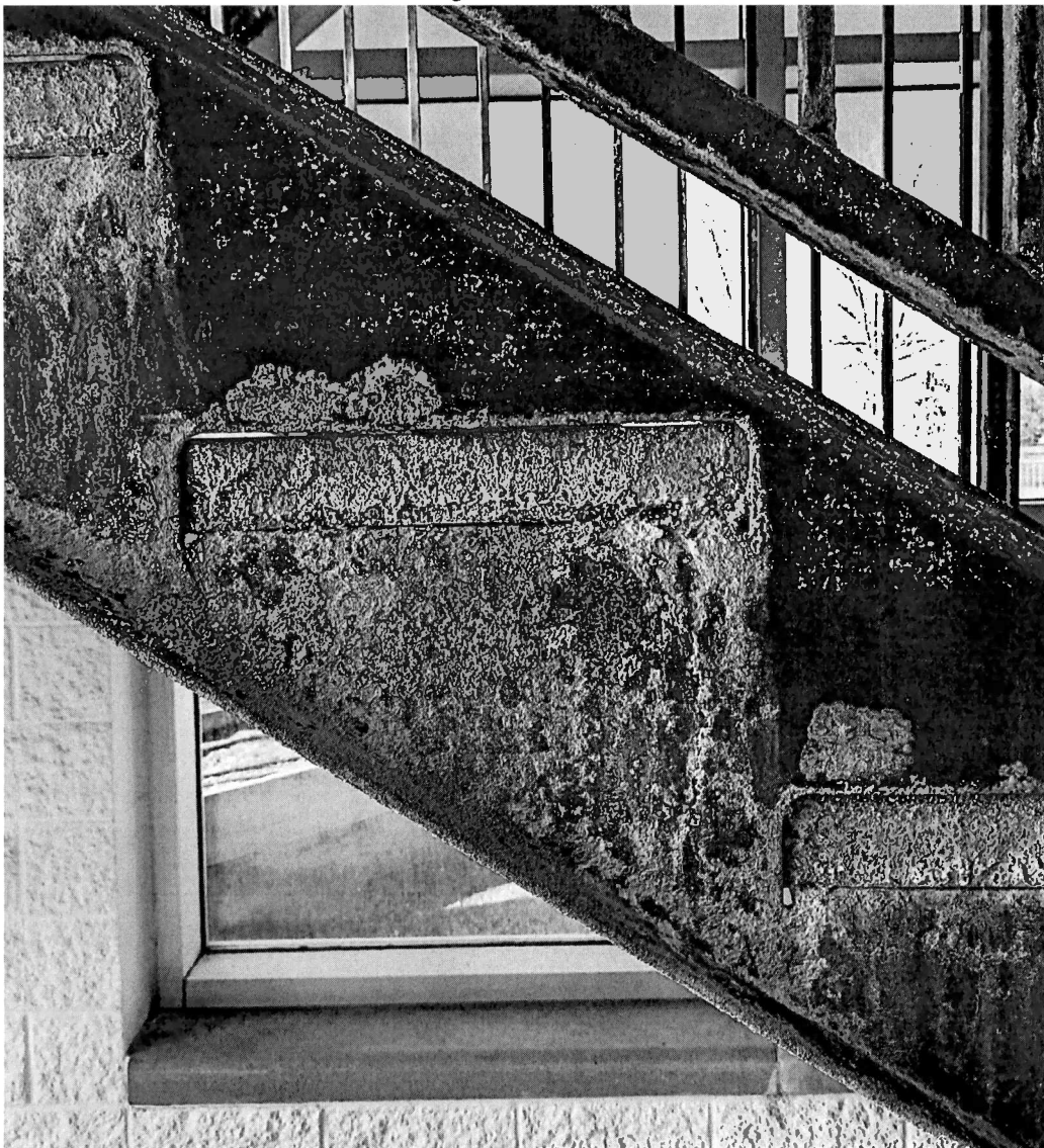
Figure 25 stairs at slide structure.
