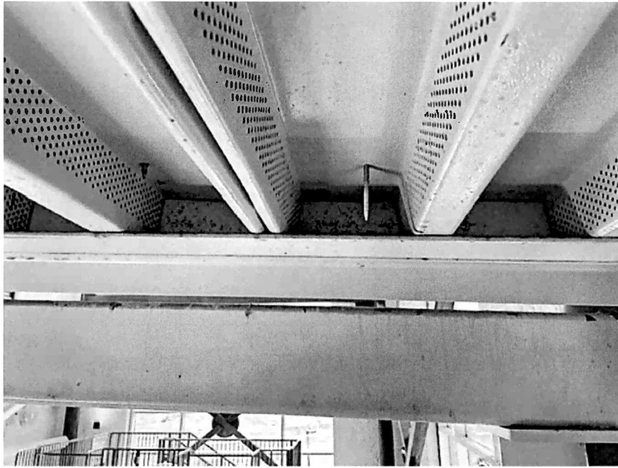
Photo-17: Undamaged roof deck bearing at west side of tower
